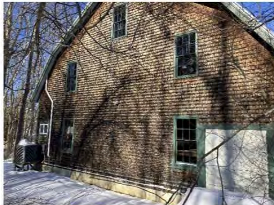
4) Exterior – West façade
